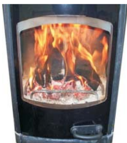
Fig.5 Fire well under way – reduce air setting to 3
